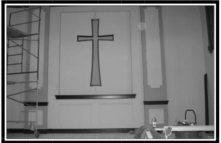
Completed sliding dossal doors with cross outline
