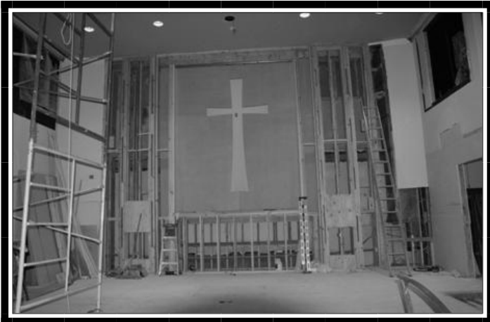
The dossal doors, framed and halfway finished
