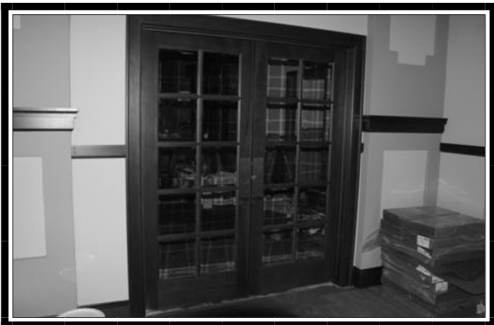
Almost completed French doors leading into the parlor from the sanctuary
